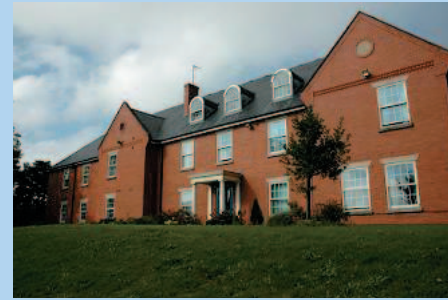
We look forward to the opening of the Hazelwood House , a PiC facility which has been completely refurbished to provide a low secure service for men with learning disabilities.
